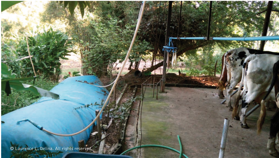
A biogas digester in Kaeng Krachan uses cow manure as a feedstock. This plastic digester is an innovation from the classic concrete-style biogas digesters.
